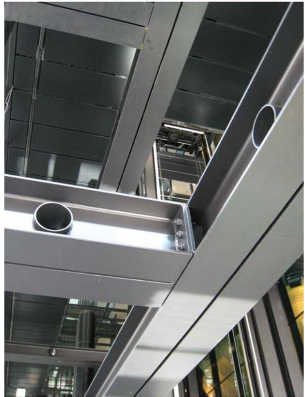
Figures 33 and 34. European Court of Justice in Luxembourg, December 2008, with outside (on the left) and inside (on the right) structural steel based on a large extent on steel columns and beams taken from the structural steel of the initial Court of Justice erected in 1972
