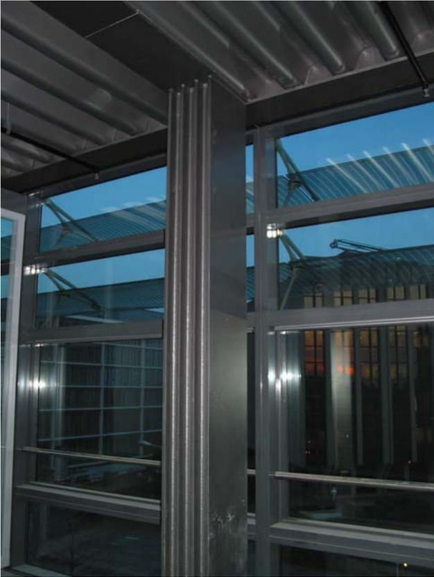
Figure 9. Chambre de Commerce with visible, unprotected steel columns supporting the composite beams
