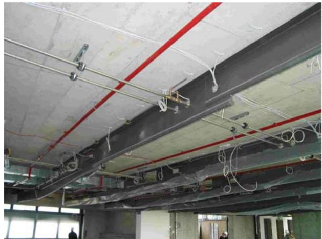
Figures 16 and 17. DEXIA-BIL building A; intermediate floor level with the visible, unprotected nine composite circular columns supporting the composite beams on the left, and with visible, unprotected composite beams on the right
