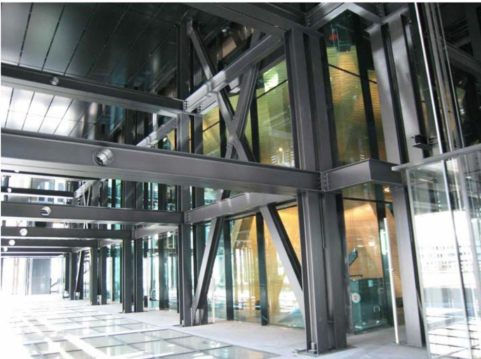
Figure 39. Two transversal wind bracings situated between levels 3 and 6, similar wind bracings have been foreseen between levels 6 and 9; as a total four transversal and four longitudinal wind bracings were erected for the central core building which covers a surface of 4070 m<sup>2</sup>
