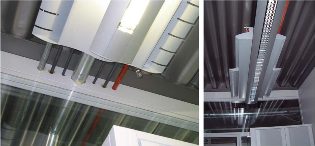
Figures 12 and 13. Lighting and air distribution units suspended from the profiled decking, also created by the late Claude Vasconi, 1940-2009
