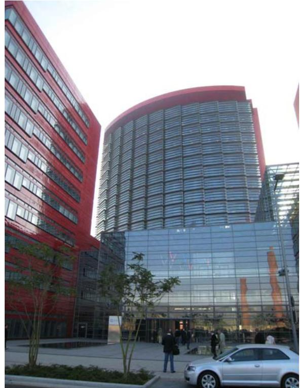
Figures 26 and 27. DEXIA-BIL tower building as finished end 2006 with enameled steel façade and in the foreground concrete columns of the former blast furnace charging device on the left, and on the right with the atrium based on a 3-D space steel truss spanning between the various buildings
