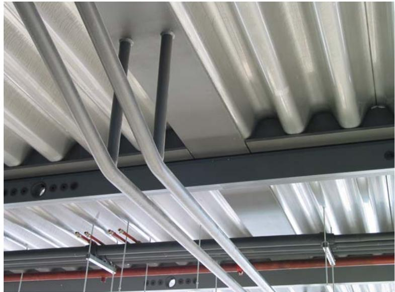
Figures 10 and 11. Tension rods sustaining the composite beams
