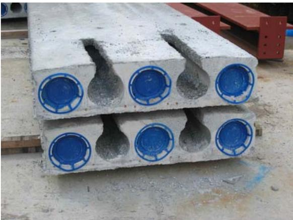
Figure 46. The correct way of preparing hollow core slabs before erection
