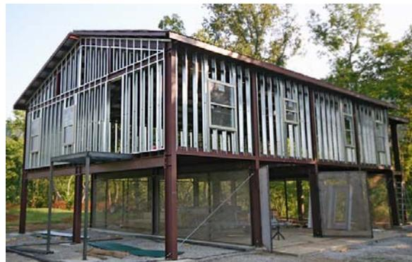
Figures 53 and 54. Prefabricated steel houses, easy to erect and with high safety level
