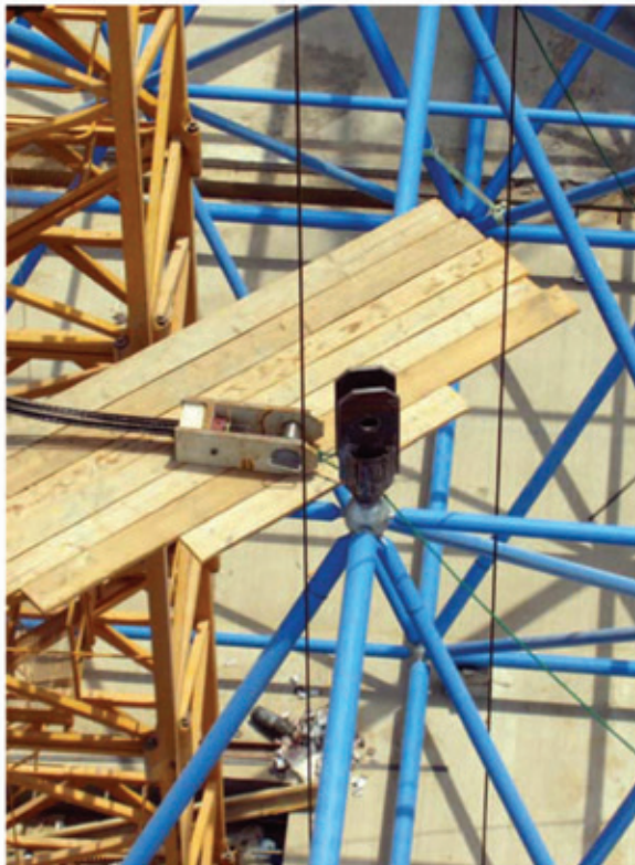
Figure 3. Lifting connection elements
