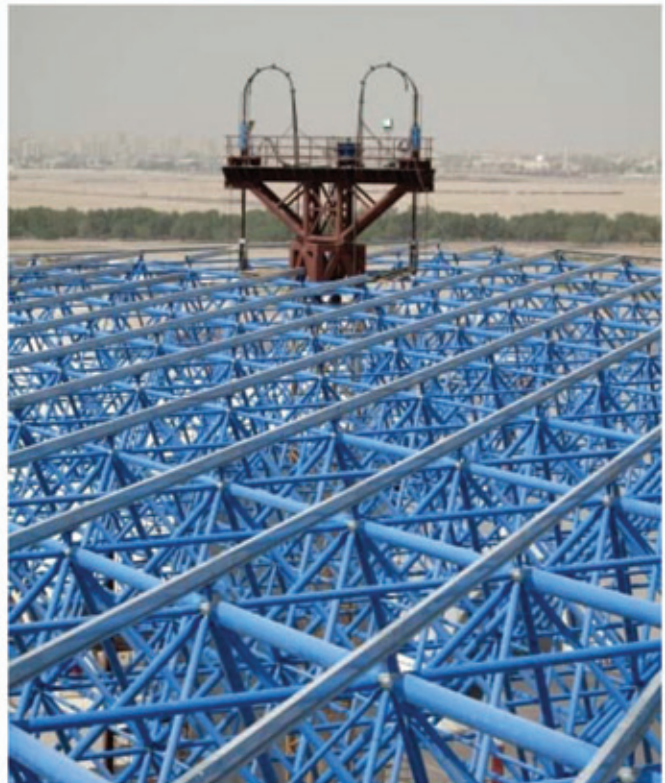
Figure 4. Lifted space frame with hydraulic jacks
