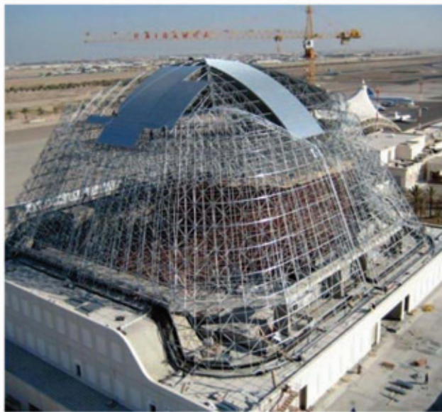
Figure 15. General view before cladding works
