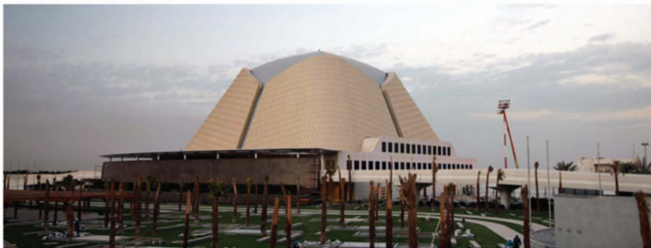
Figure 19. General outside view of the amiry terminal after completion of cladding works
