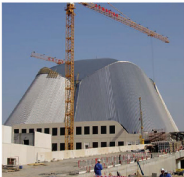
Figure17.General view after first layer of cladding
