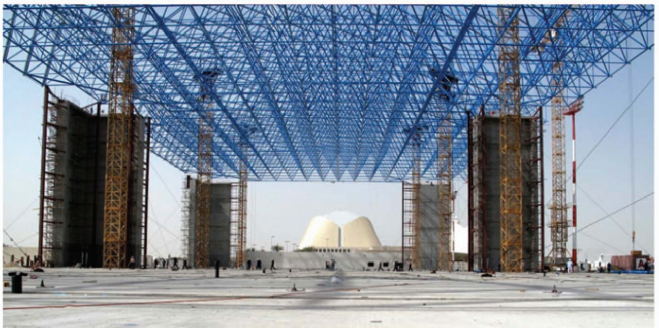
Figure 8. View of the airbus a380 hangar during installation after lifting process
