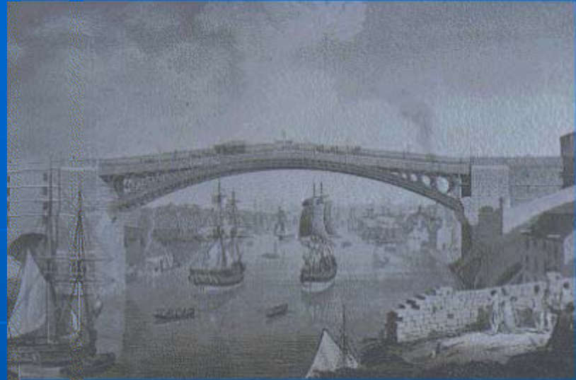
Thomas Wilson's Wear Bridge
